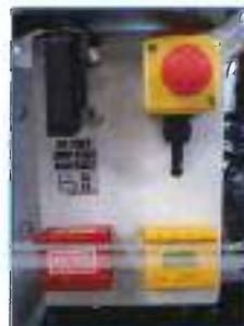
Battery isolation switch located on the control panel at the front right hand side of the module
